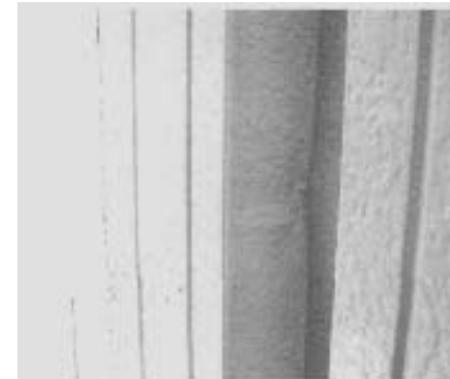
Typical local indentation of interior surface from strike on exterior surface (9-pound 2x4 at 35 mph)
